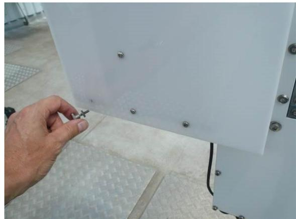
**Fig.2.6.4: Remove heater mounting screws from the blower.**
