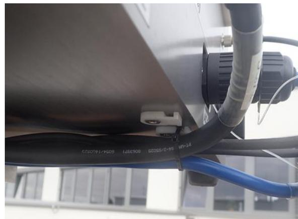
**Fig.2.5.9: Fastening cables on the radiometer's bottom plate.**
